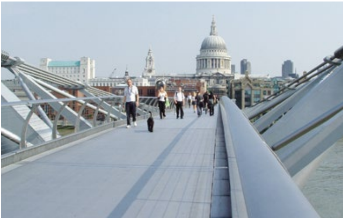
Millennium Bridge, London, GB
