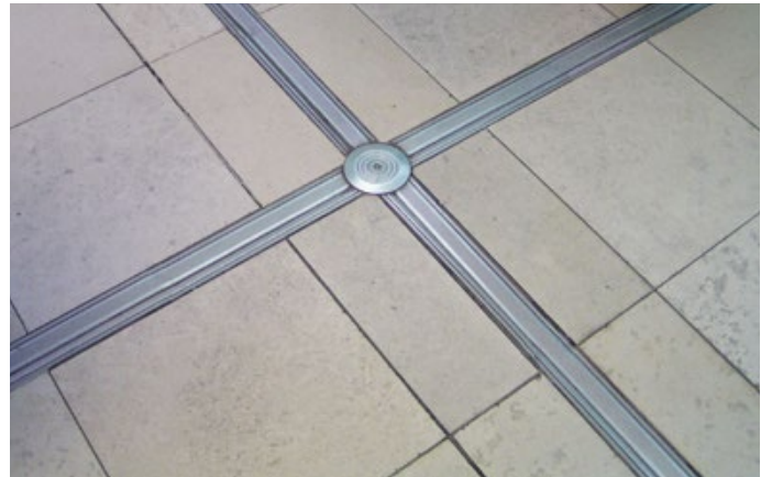
City Centre Halle shopping centre
