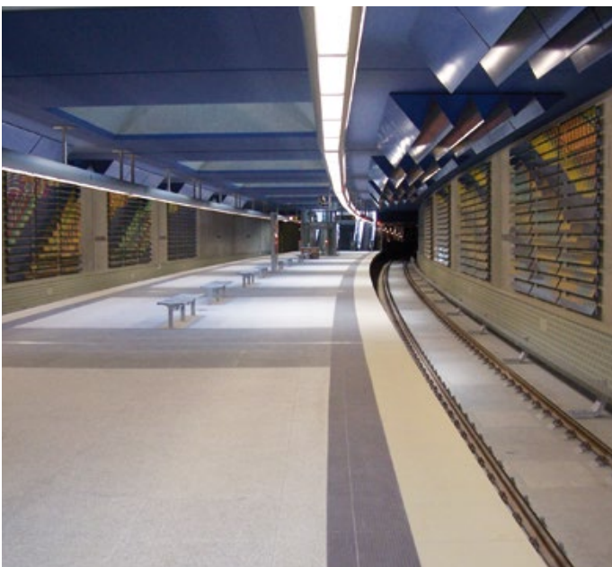
Hamburg airport, underground
