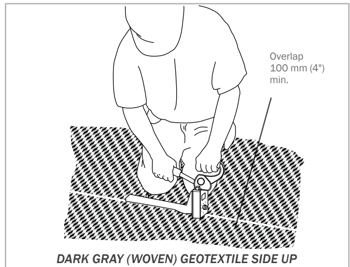
Figure 1.2 - Secure overlaps together with fasteners
