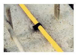
Alternatively, the hose can be fastened in place with plastic clips, either set in the fresh concrete or subsequently hammered into an 8 mm drill hole.
