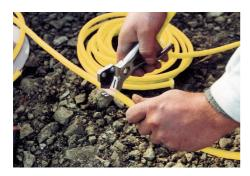
The product is supplied on a 100 m reel. Use a suitably sharp tool to cut the hose to the required length.
