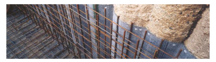
nstall VOLTEX® GB-500 waterproofing membrane composite with the bentonite side against the concrete wall on cast-in-place concrete foundation walls prior to backfilling. VOLTEX® GB-500 waterproofing membrane composite may be applied as soon as the forms are removed. It is not necessary to wait for the concrete to completely cure. Use VOLTEX® GB-500 waterproofing membrane composite with concrete cast with conventional forms that produce smooth surface.
