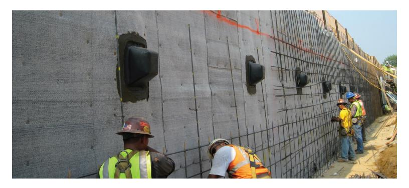
nstall VOLTEX® GB-500 waterproofing membrane composite with geotextile side against the cast-in-place concrete foundation walls prior to backfilling. VOLTEX® GB-500 waterproofing membrane composite may be applied as soon as the forms are removed. It is not necessary to wait for the concrete to completely cure. Use VOLTEX® GB-500 waterproofing membrane composite with concrete cast with conventional forms that produce smooth surface.
